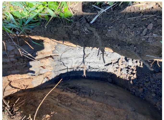
Photo No. 12: View of Test Pit 12.
