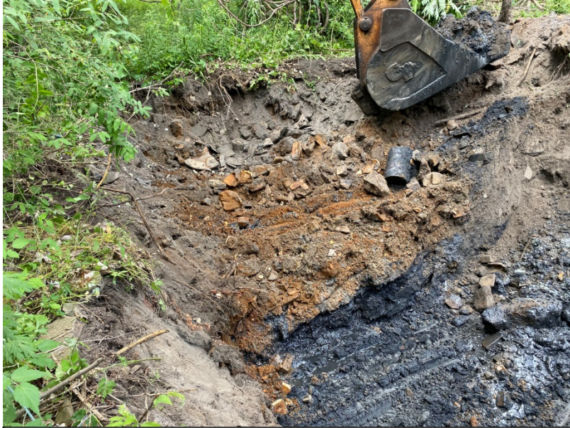
Photo No. 17: View of Test Pit 15.
