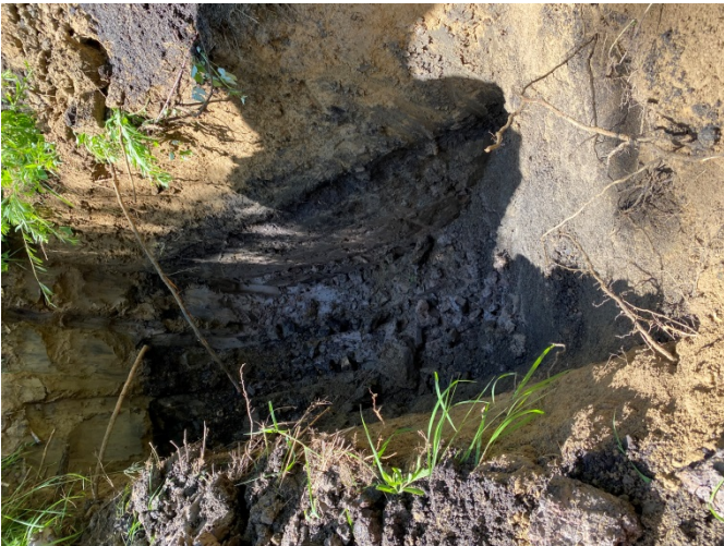
Photo No. 3: View of Test Pit 3.
