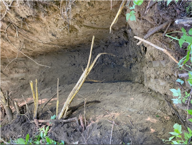
Photo No. 1: View of Test Pit 1.
